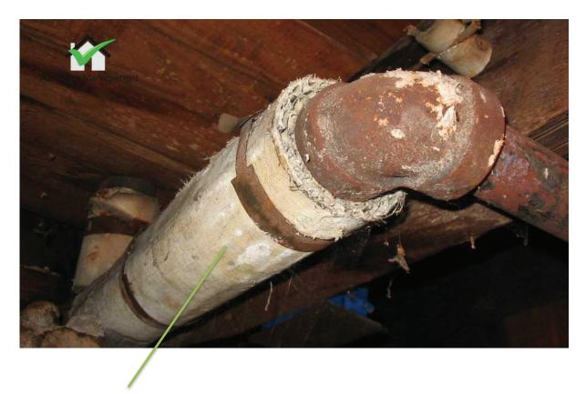
Example of lagging around a heating pipe system in a commercial building
